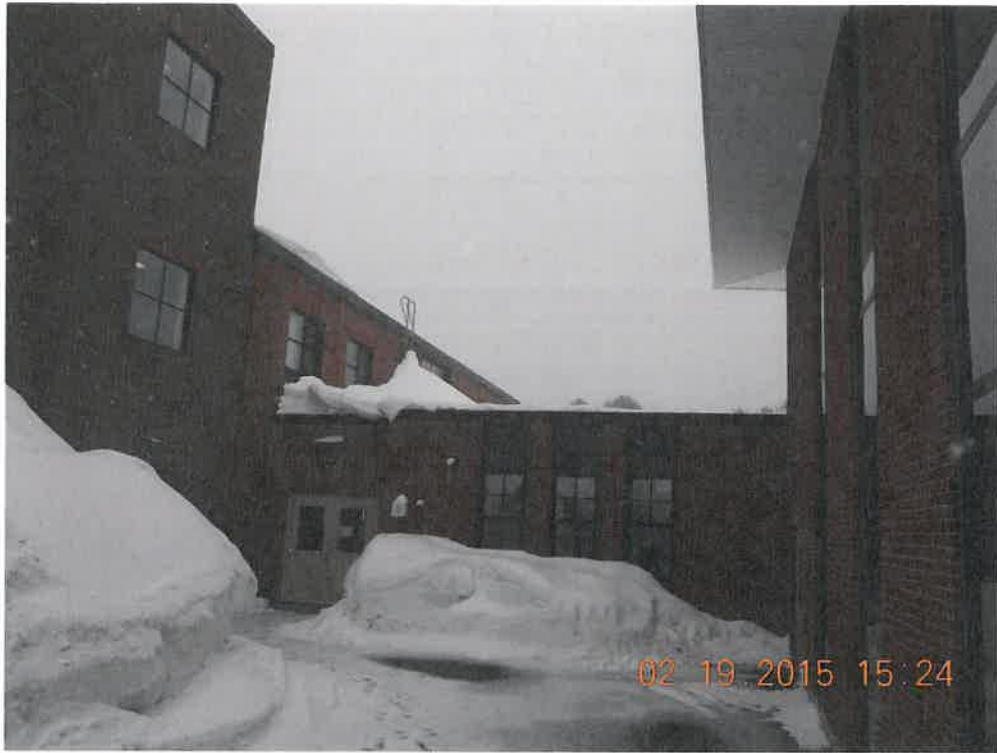
Build up of snow on low roof above corridor
