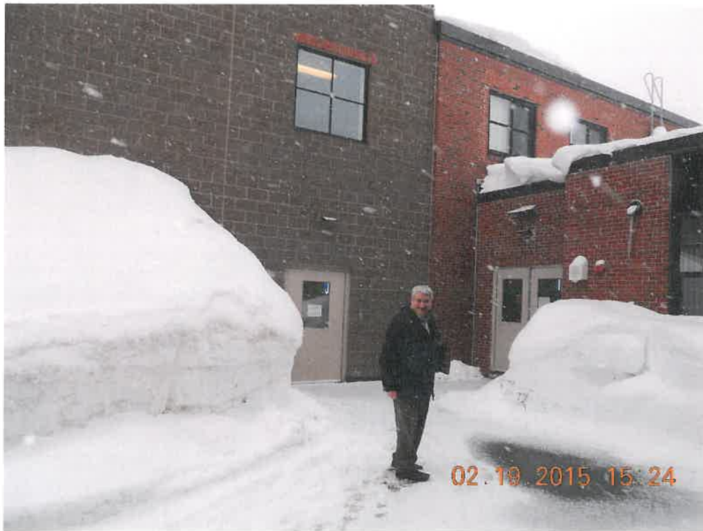
Build up of snow on low roof above corridor
