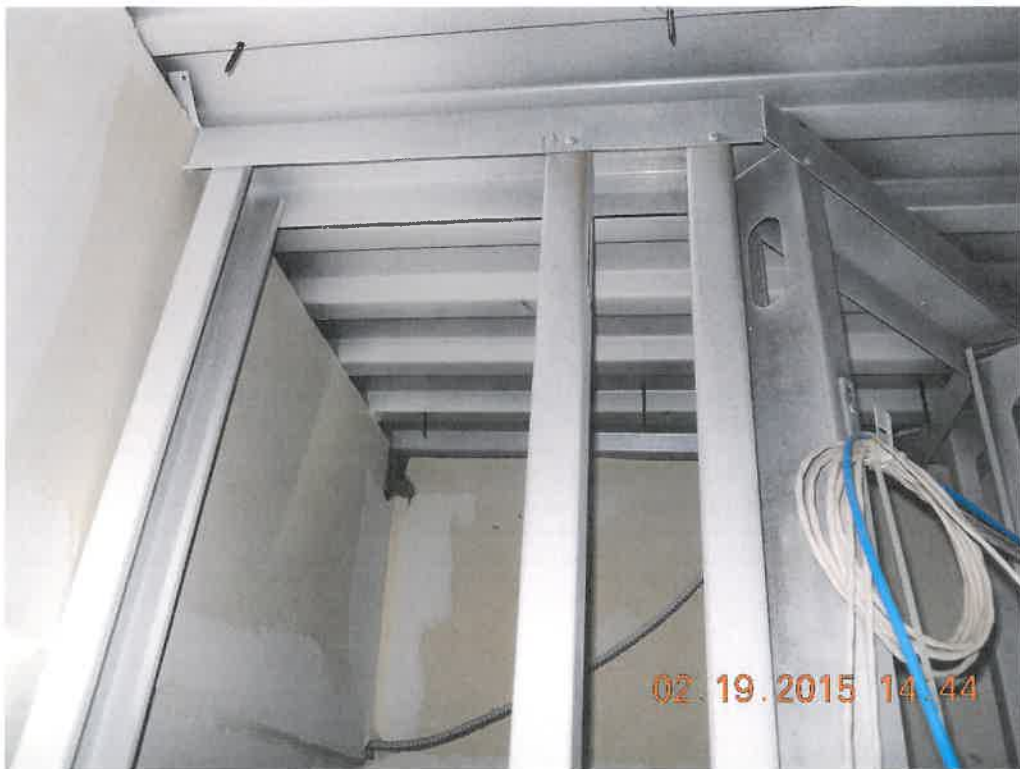
Stud wall attached directly to roof deck.
