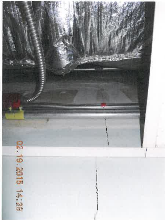
Corridor wall near room T308 / T307. Failed drywall joint.
