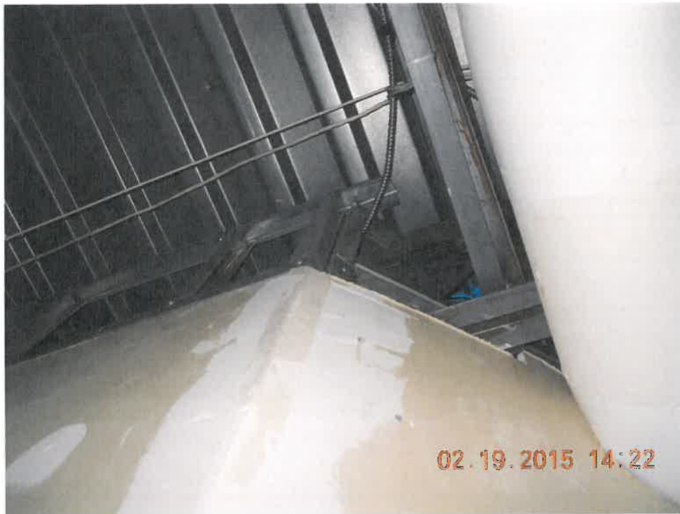
Studs extend to roof deck. No deflection track.
