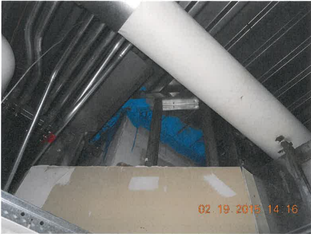
Studs attached directly to roof deck
