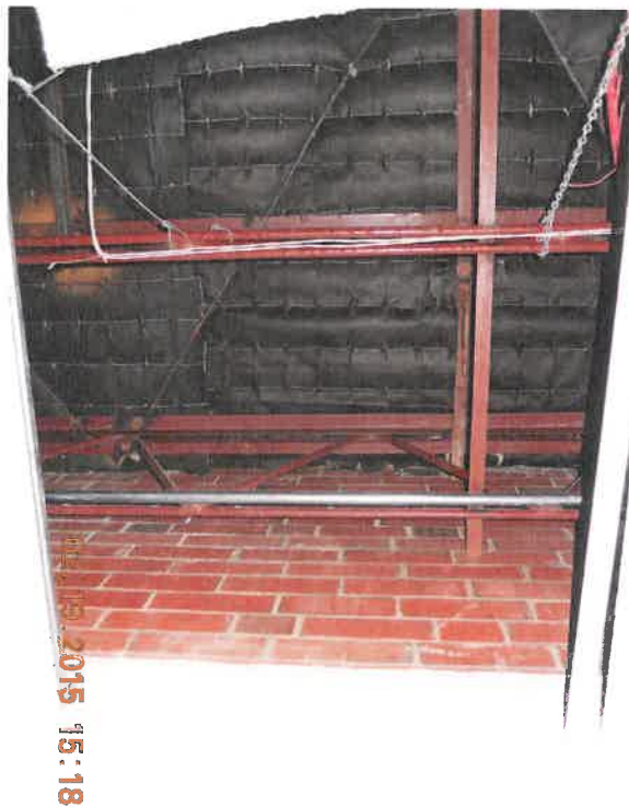
Above corridor near exterior exit. Near C124A
