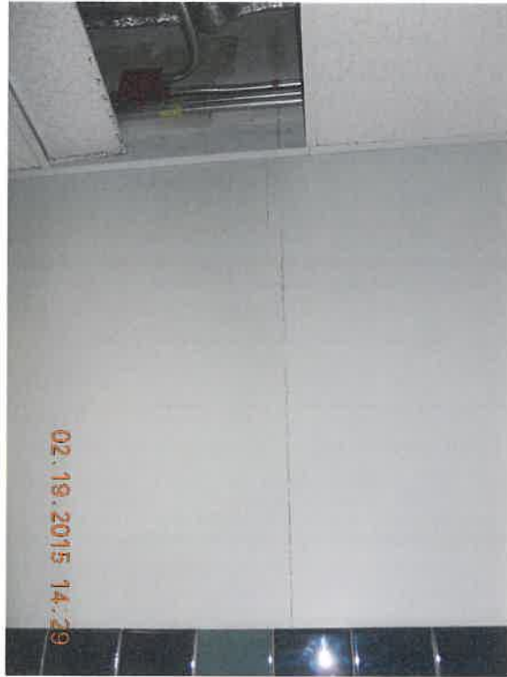
Corridor wall near room T308 / T307. Failed drywall joint.
