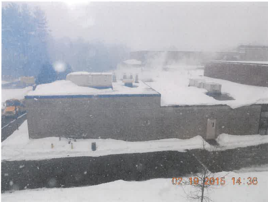
Roof top view
